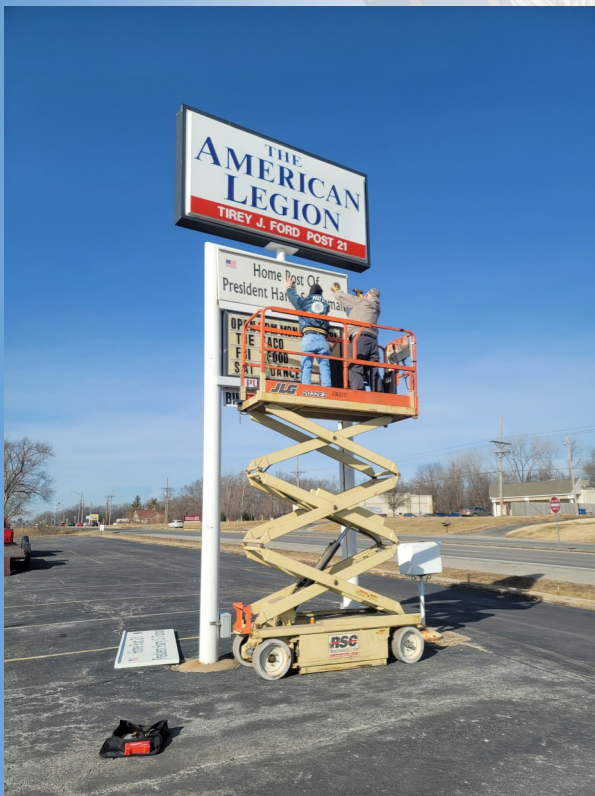
Randy Bray and George McCorkendale installing the finished signs
